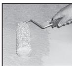
**Step Two:** Roll on a second coat with the same roller in the opposite direction. This will fill imperfections from the first application and make the surface look uniformly solid and stone-like. You can use the same color as the first coat – or go with a different color altogether for an attractive multi-toned texture.
