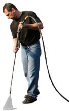
loose concrete by holding the spray tip a few inches from the surface using a slow back and forth sweeping motion across the surface at a rate of approximately 100 sq. ft. per 20-30 minutes.
