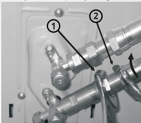
4. Then, tighten the connector slightly beyond that point to apply torque to the connector. Please refer to the manual for information about torque requirements. Repeat the same steps for the top screw connector.
