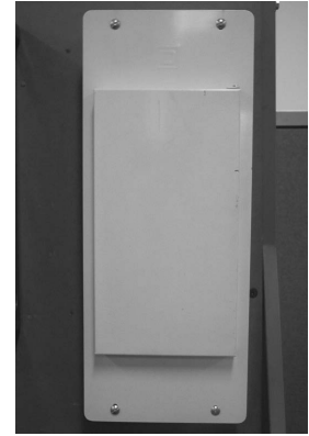
Step #4 Complete Installation
