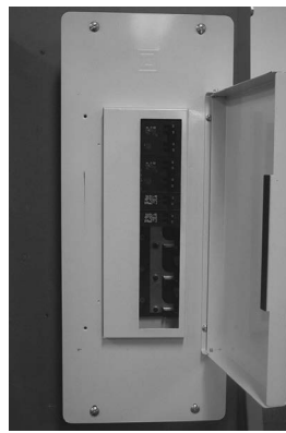
Step #3 Install New HFLCI
