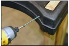
5. Drill 1 screw into each section, through the wood. On the corners, make sure to drill on an angle. Do not overtighten.
