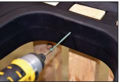
5. From the under side of the seat, drill 1 screw into each section, through the wood. On the corners, make sure to drill on an angle. Do not overtighten.
