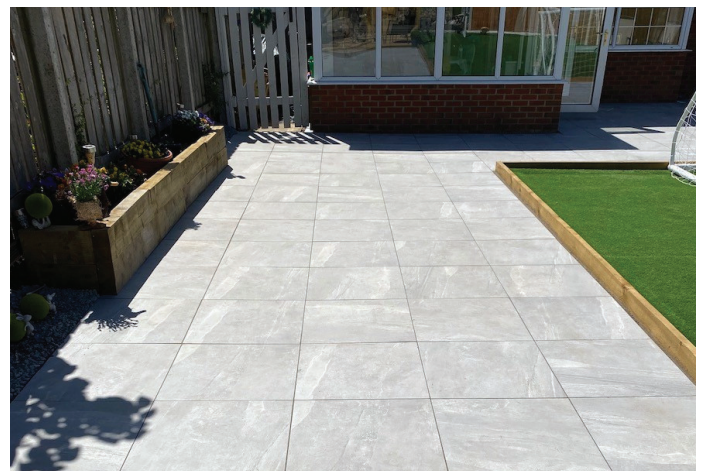
Porcelain Tile Patio and Walkway
