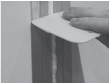
FIGURE 18: REMOVING EXCESS SEALANT
