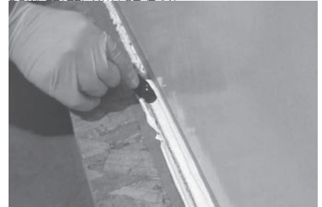
FIGURE 23: HORIZONTAL FINISH WITH ROUNDED CORNER
