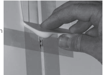
FIGURE 17: APPLYING THE PAINTER TAPE HORIZONTAL IN 3' SECTIONS
