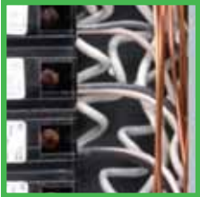
Pigtail Neutral Connections
