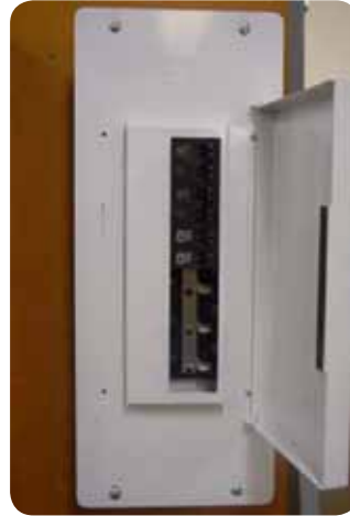
Step #3 Install New HFLCI
