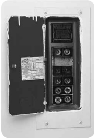
Step #1 Identify Box Dimensions and Catalogue Number
