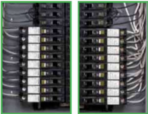
Plug-on Neutral Connections
